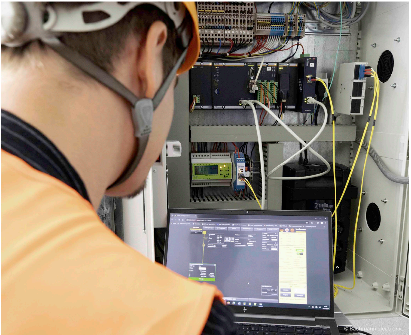
Remote access to a visualisation allows topologies, signal flows, diagrams and set values to be displayed via an internet browser
