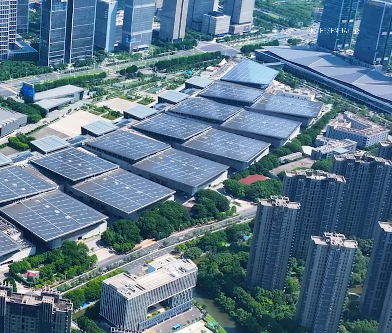
25 MW Microinverter powered project, Nanjing, China
